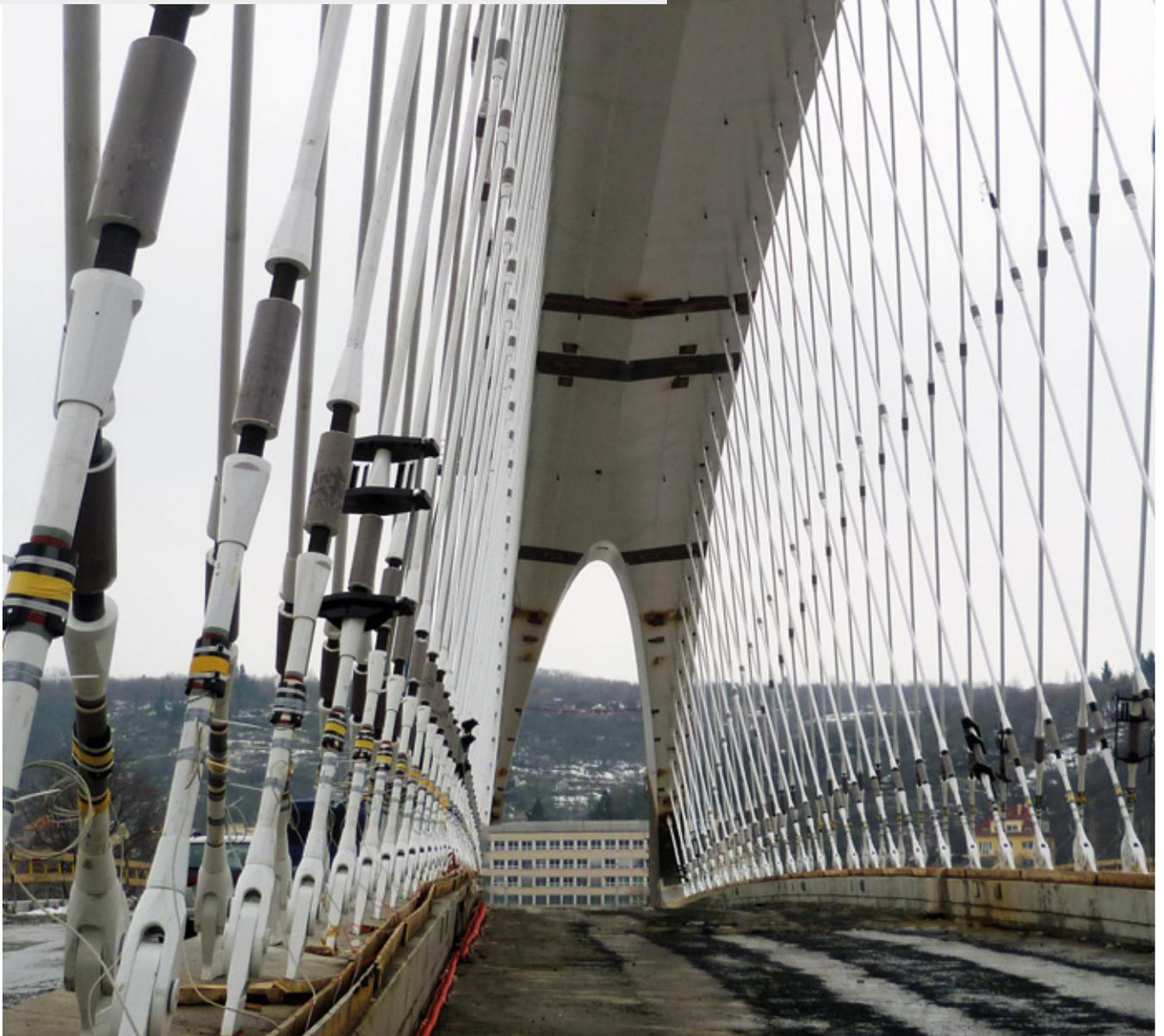
**PONT SCHUMANN** – This two arched stainless steel road and pedestrian bridge in Lyon France opened in 2014 and was designed by Flint and Neil. The carbon steel tendons are designed to support the feature triangular arch sections of stainless steel. The designer required 100% X-Rays on ALL components, normalised bar material and spherical bearings throughout.
